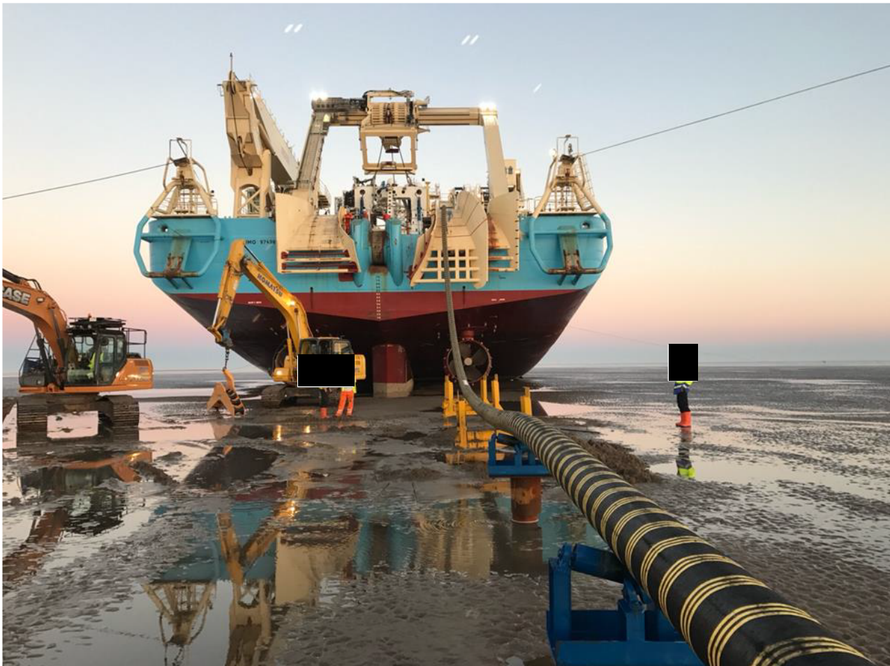
Plate 4.2 Example of cable being pulled ashore from a beached CLB (Walney Extension Offshore Wind Farm)
